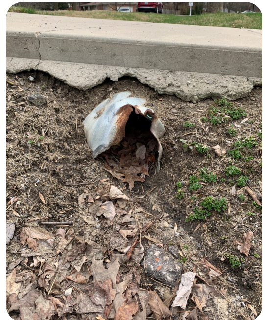
Damaged storm sewer culvert (Giffels Webster, 2020)
